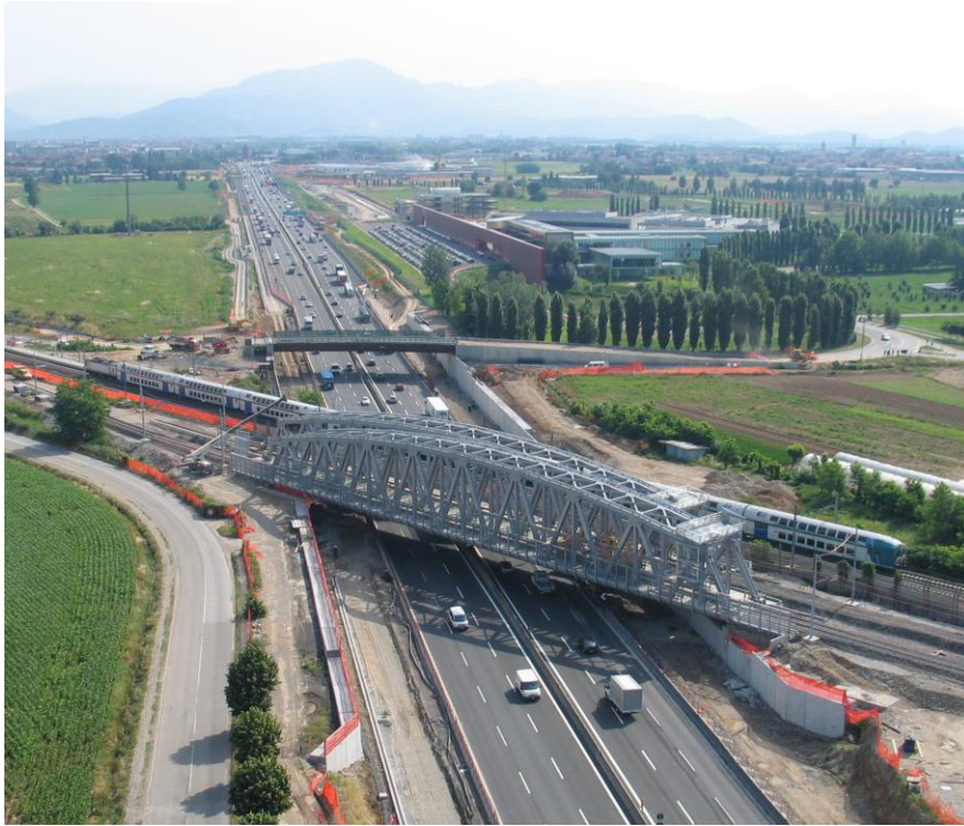
Figure 4.11.1 – View of the twin railway bridges.
